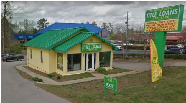
This building does not meet Standard j.
